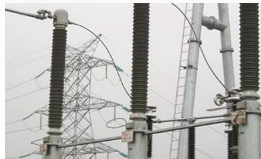
Figure 3: PCS-9250 series ECT/EVT for AIS application
