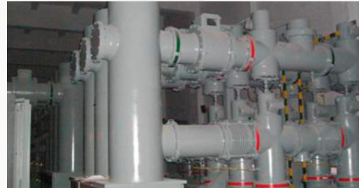
Figure 3: PCS-9250 series ECT/EVT for GIS application
