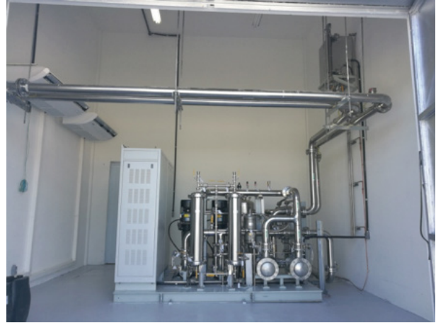
Onsite water cooling system
