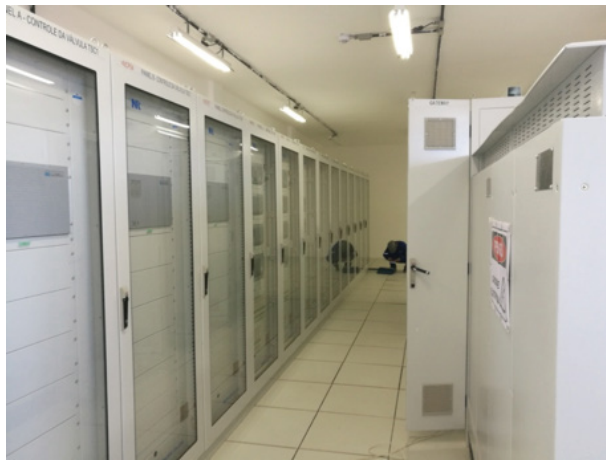
On-site protection & control panels
