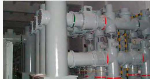
Figure 3: PCS-9250 series ECT/EVT for GIS application
