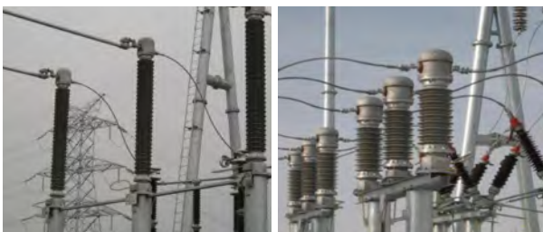
Figure. PCS-9250 AIS ECT/EVT in a 220kV digital substation in Heilongjiang Province
