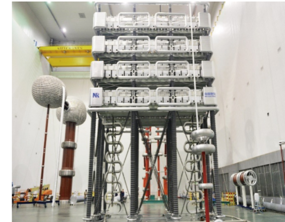
\pm 535 kV/3000 MW converter tower
