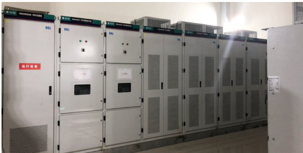
Static frequency converter picture taken on site
