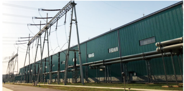
Outdoor picture of synchronous condenser on site
