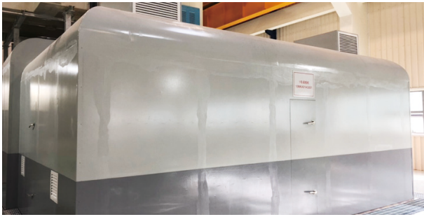
Synchronous condenser picture taken on site
