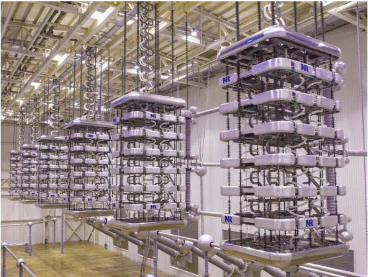
Figure 2 ±800kV Converter Valve Hall
