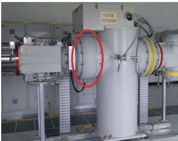
Figure 2 Optical CT in GIS Application
