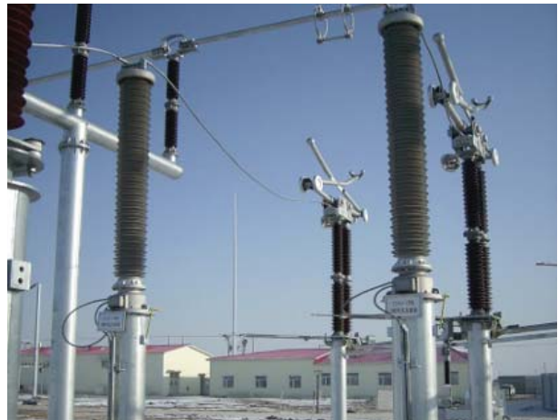
Figure 4 Electronic VT in AIS Application
