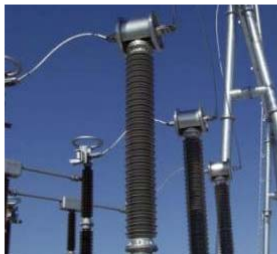
Figure 5 Optical CT in AIS Application
