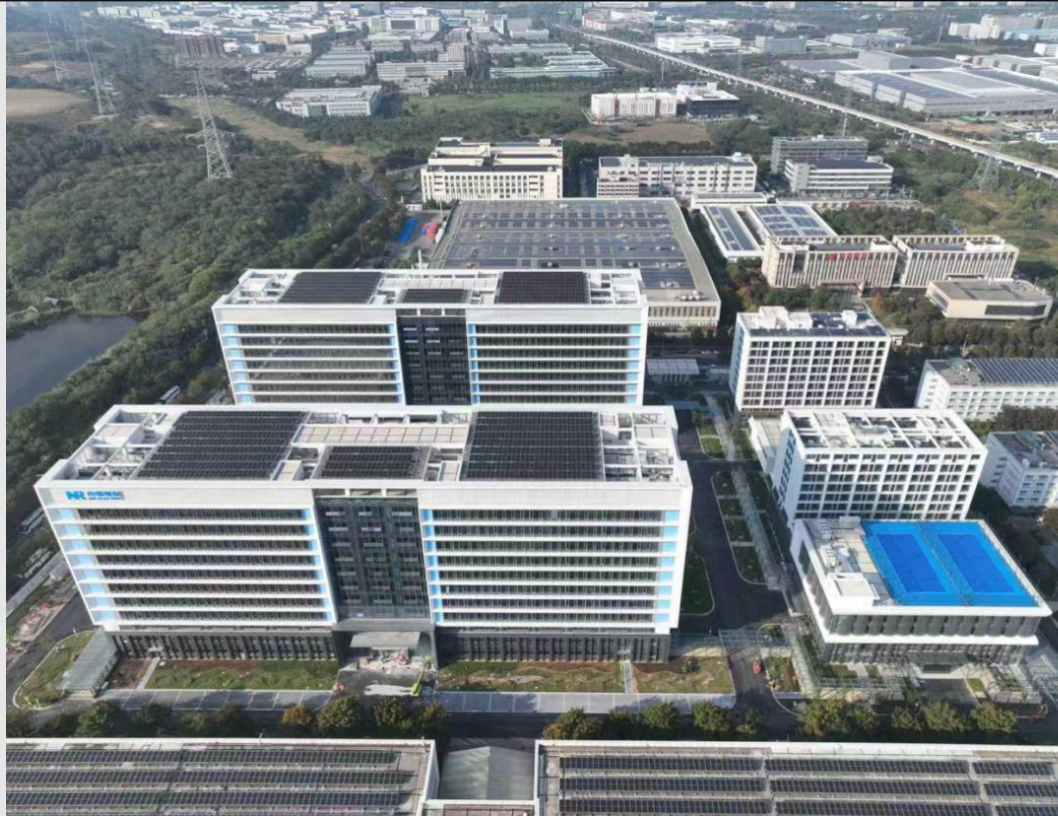
Aerial View of the Jiangjun Road Phase II Rooftop Solar Water Heating System
